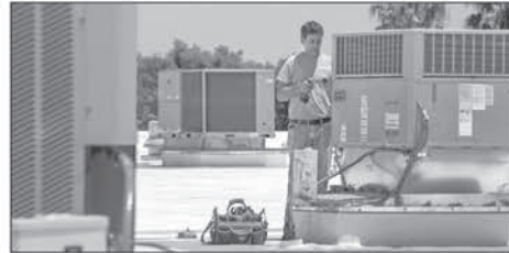
AIR CONDITIONING INSTALLS
