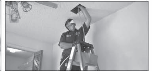
AIR CONDITIONING DUCT CLEANING
